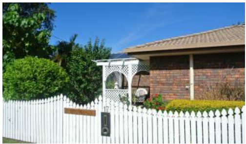
17 Springdale Street, Rothwell
