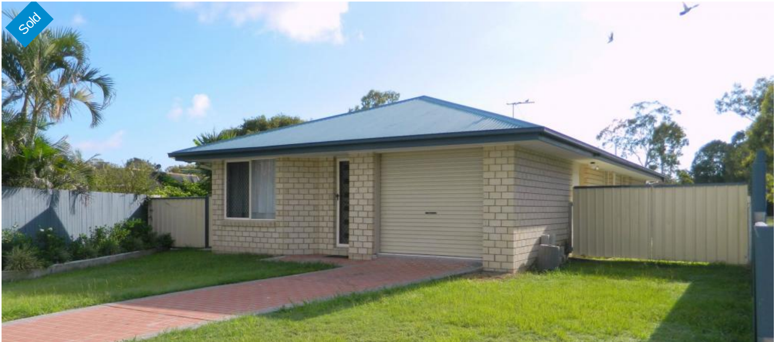
3 Aberfoyle Drive, Deception Bay
