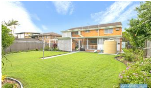
125 King St, Woody Point
