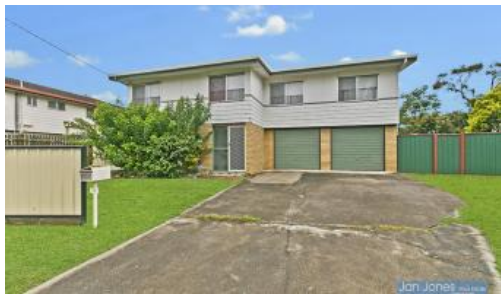
4 Breavington Ct, Deception Bay
