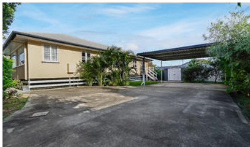
17A Collins Street, Woody Point
