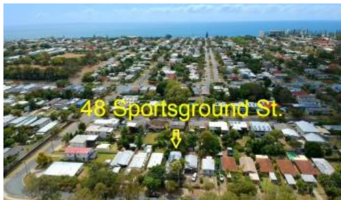
48 Sportsground St, Redcliffe
