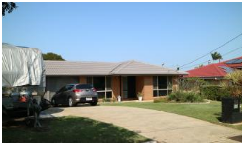
121 King St, Woody Point
